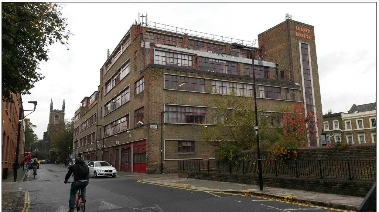
Photograph 3: existing building (Henshall Street and Dove Road elevations, with St Paul's Church in the background)
