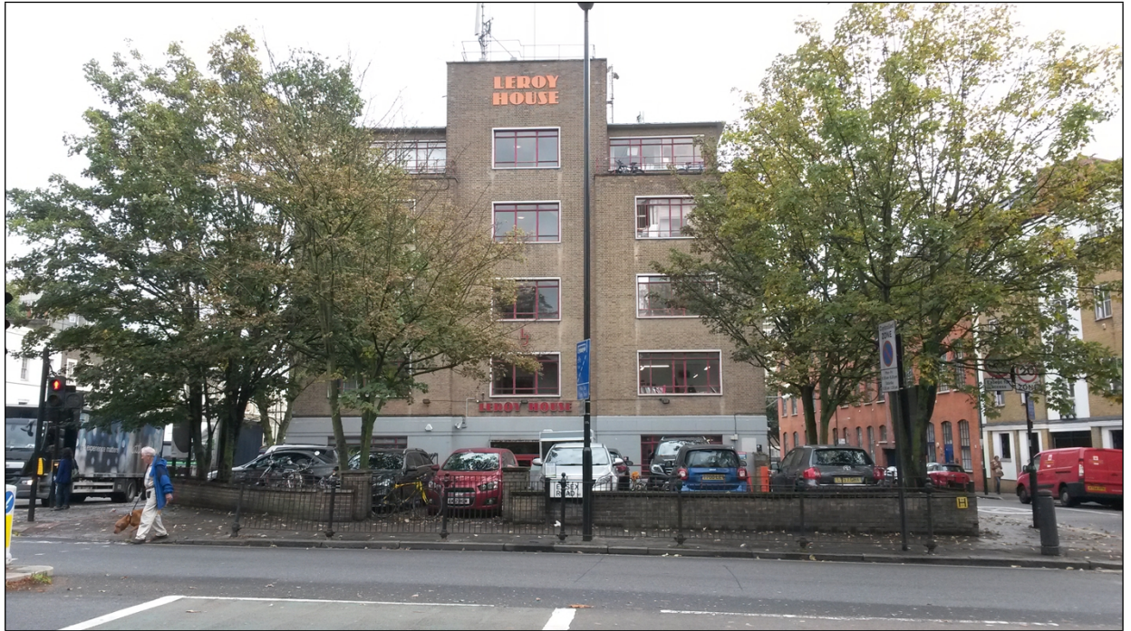
Photograph 2: existing building (Essex Road elevation)
